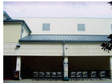
Bracket Supported Roofed Entry Pediment with Cornice and Cornice Molding Flat Roof and Pitched Roof Combination
