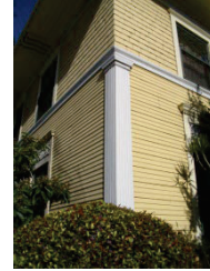
Classical Entablature Entablature (examples) Building Corner Trim
