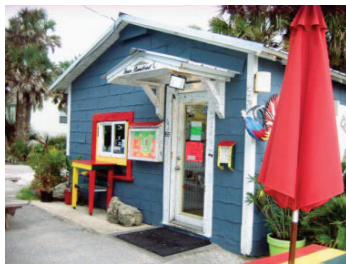
Bracket Supported Roofed Entry Pediment with Cornice and Cornice Molding Flat Roof and Pitched Roof Combination
