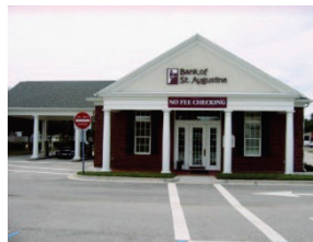
Bracket Supported Roofed Entry Pediment with Cornice and Cornice Molding Flat Roof and Pitched Roof Combination
